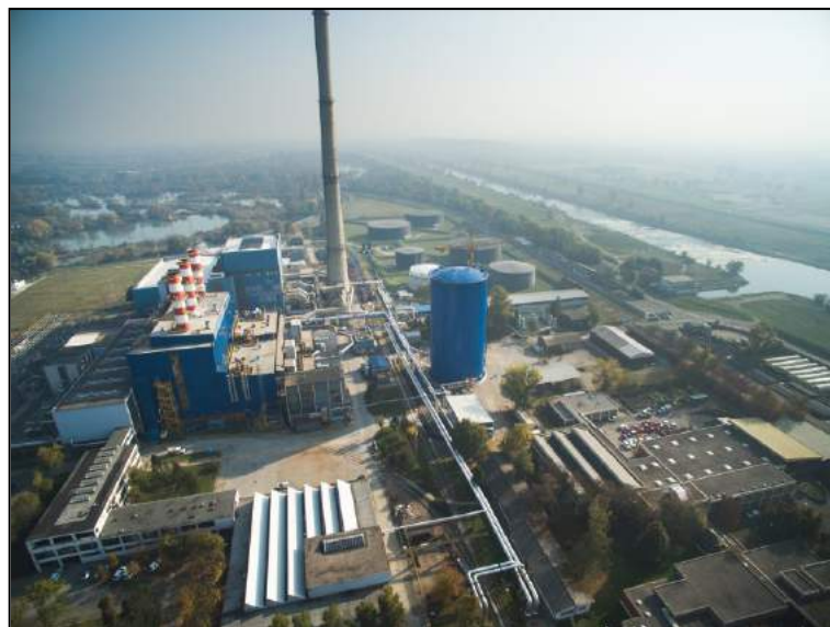
Sl. 1.2-2: Akumulator topline u TE-TO Zagreb
